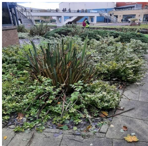
Photo 2: Slate planters in the east section of the site.
